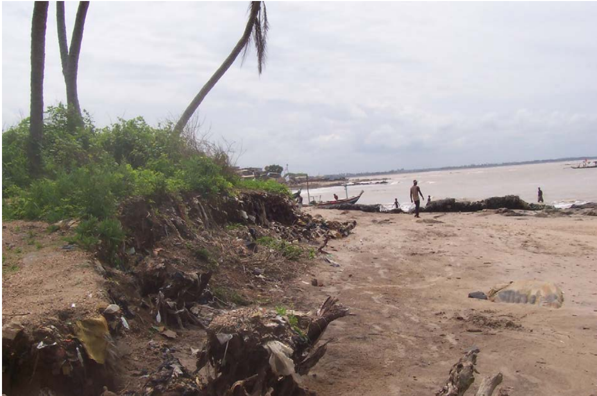
Plate 15ii: Effects of Sea Erosion at Aboesi
