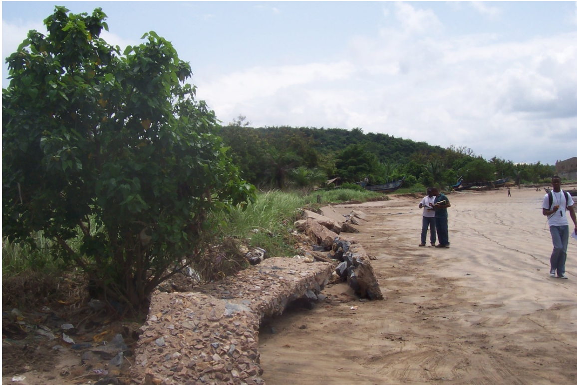
Plate 8 i: Shama Collapsed Sea Defence Wall
