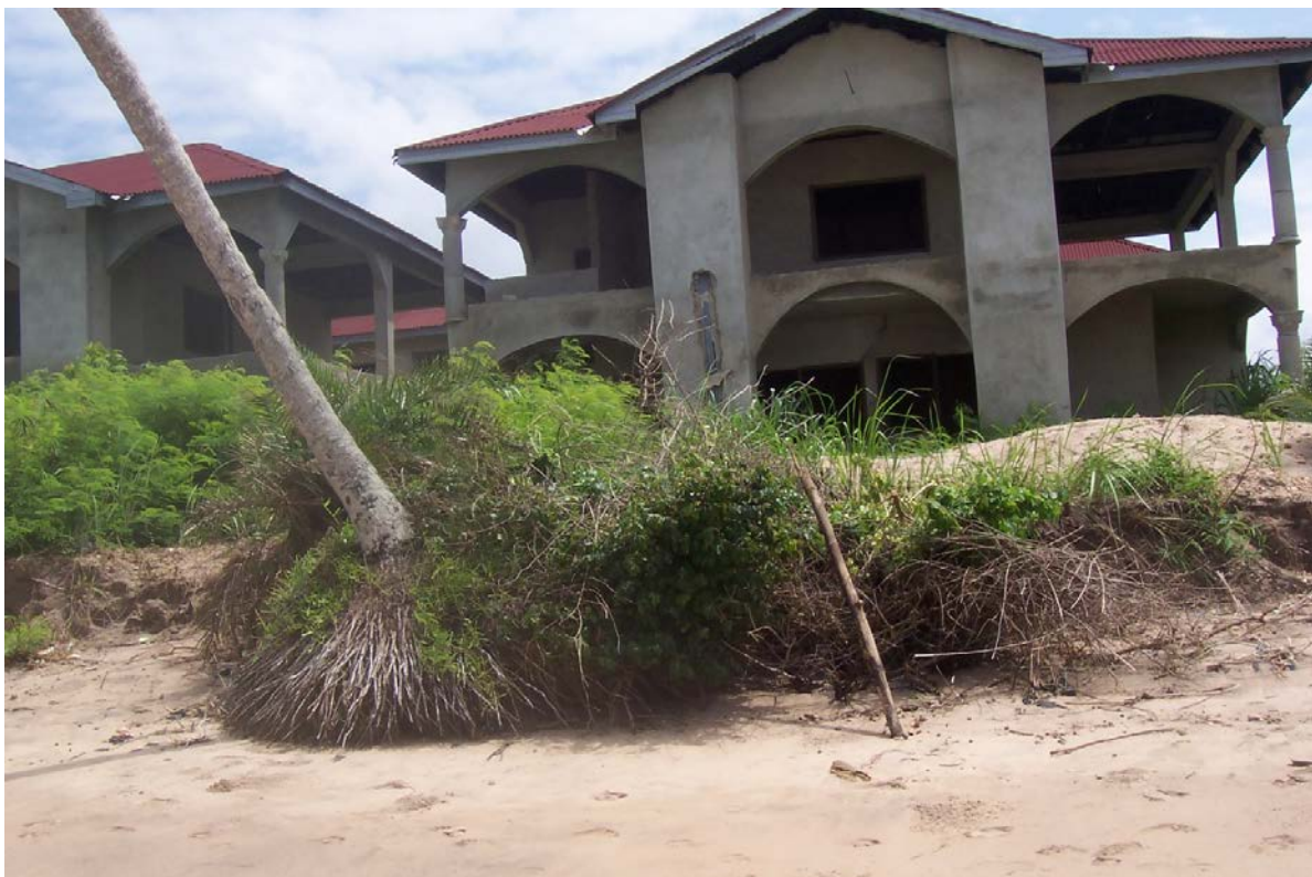
Plate 11: Built-Up area close to Shama Beach
