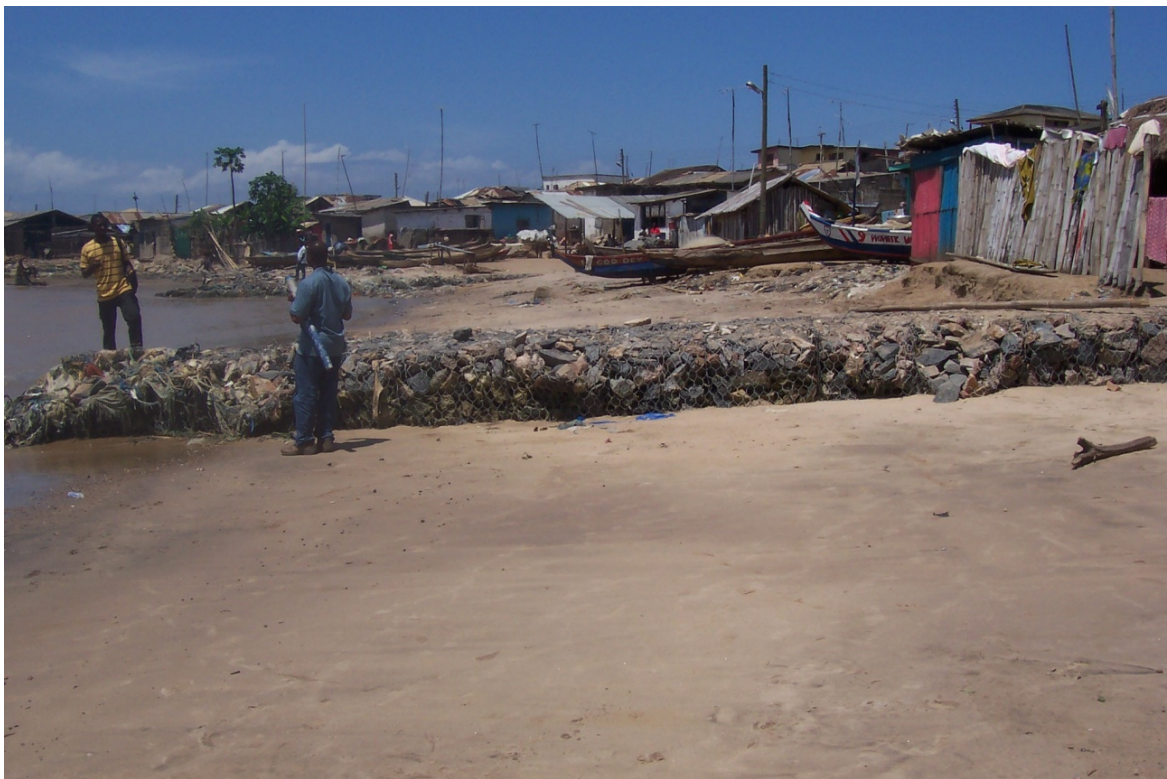
Plate 7 i: Shama Sea Defence Wall
