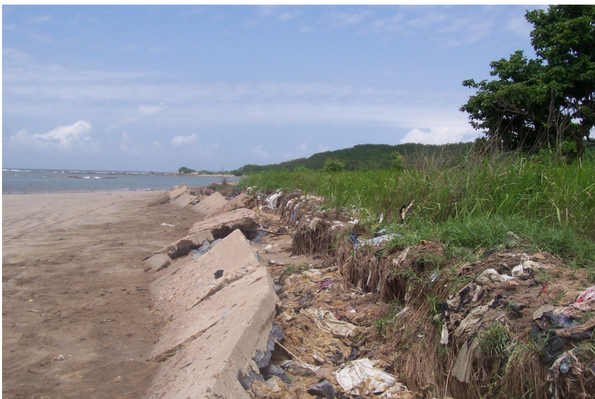
Plate 8 ii: Shama Collapsed Sea Defence Wall
